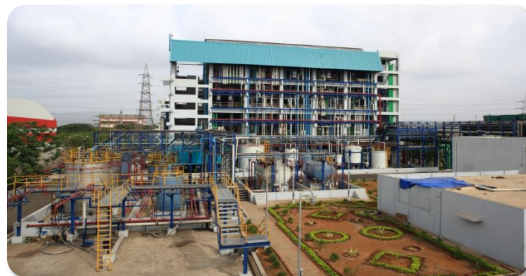
Agro Chemical Facility - Talaja
